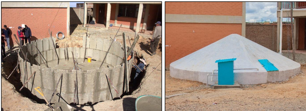
Figure 20. Left: Water harvester in construction. Right: Water harvester finalized
